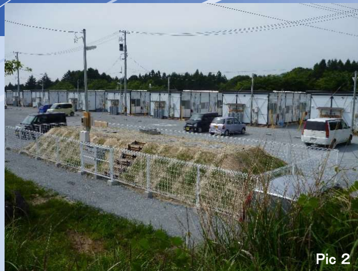
Fukushima Prefecture (Semi-underground installation + embankment: 45 EP × 2 units)
