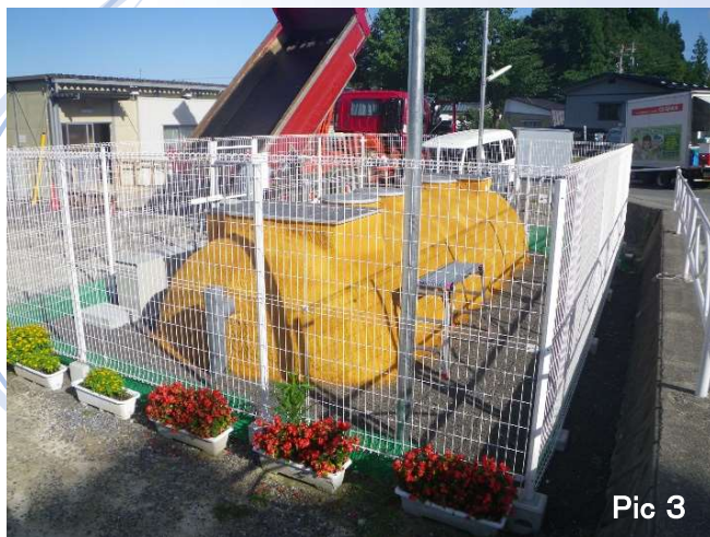
Iwate Prefecture (Semi-underground installation, heat retention measures : 42 PE)
