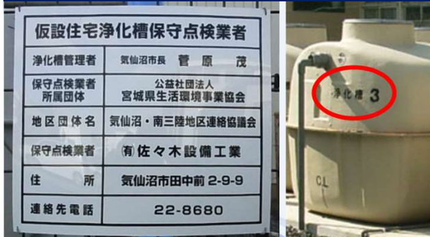
improvement approach for maintenance (sign boards and numbering)
