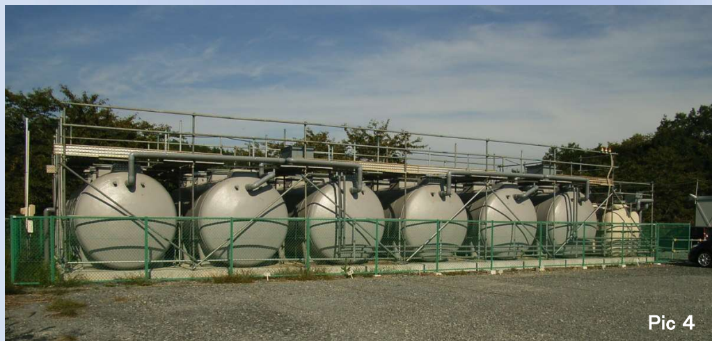
Iwate Prefecture (Ground installation, No heat retention measures: 90 PE × 6 units + 30 PE)
