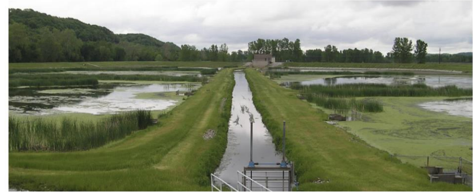
Constructed wetlands as part of the wastewater treatment
