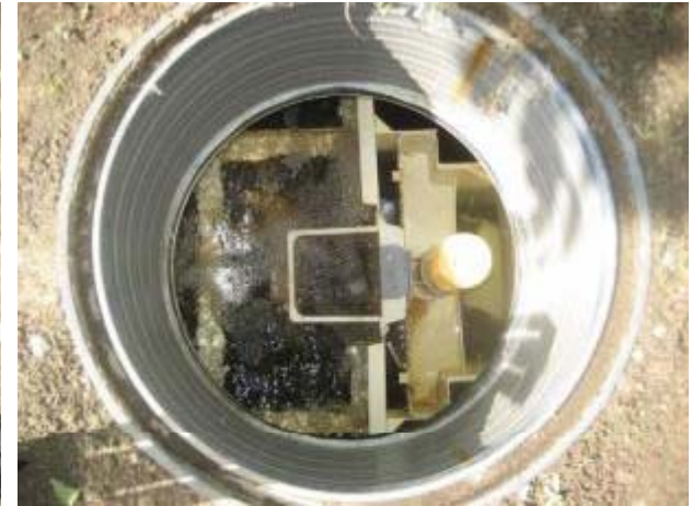
Aerobic tank and disinfection tank
