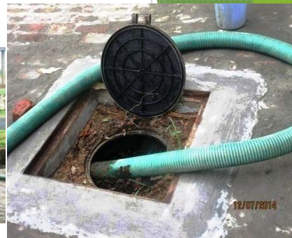
Desludging of system
