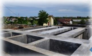
Bak Penangkap Pasir (Grit Chamber)
