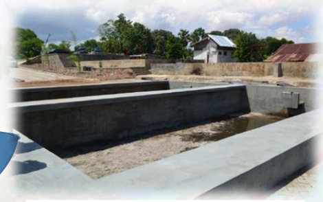
Sludge Drying Bed (SDB)
