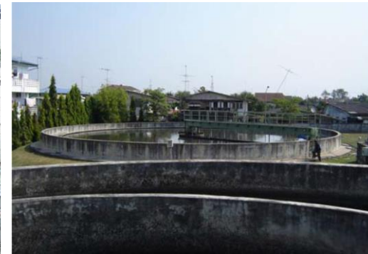
WWTP , Chachoengsao province
