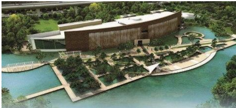
Bangsue WWTP , Bangkok
