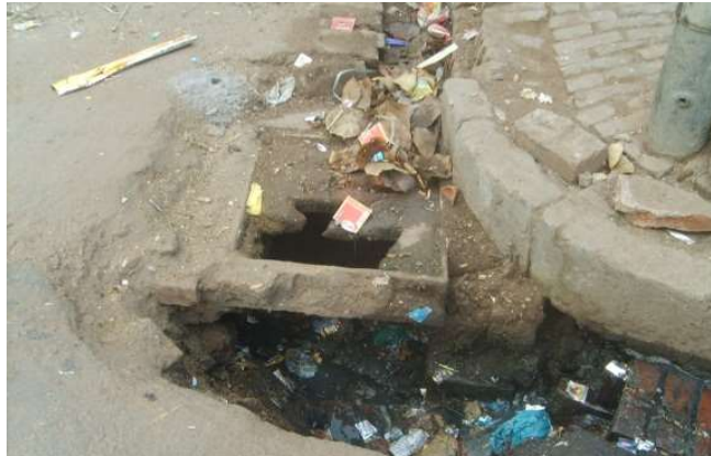
Broken gully pit
