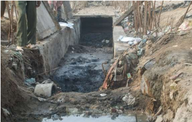
Siltation leading to clogging
