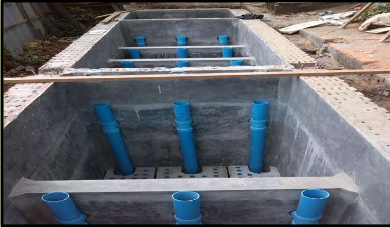
(BORDA) Decentralization Wastewater Treatment System (7m 3 /day) at B.E.H.S (1) Tamwe, Yangon
