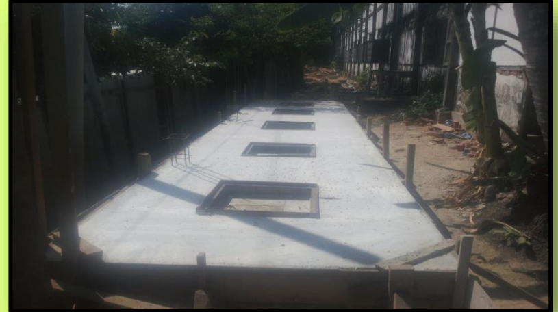
(BORDA) Decentralization Wastewater Treatment System (7m 3 /day) at B.E.H.S (1) Tamwe, Yangon
