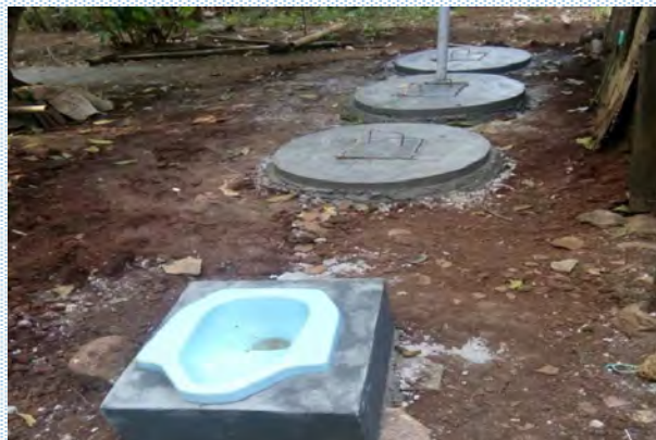
Silinder Septic Tank Construction
