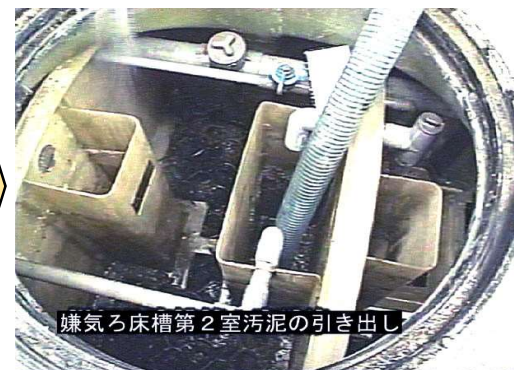
Drawing sludge out of the 2 nd -room of anaerobic filter tank
