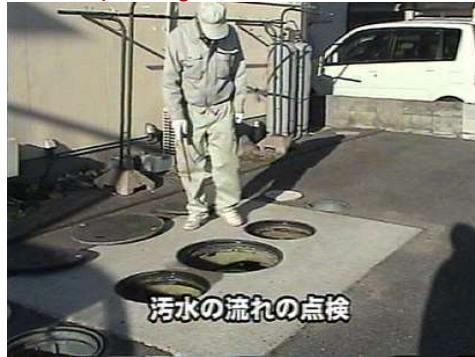
Inspecting wastewater flow
