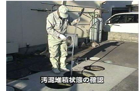
Measuring deposited sludge
