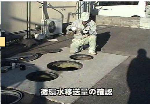
Measuring circulating water volume
