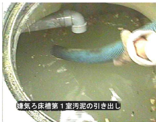
Drawing sludge out of the 1 st -room of anaerobic filter tank
