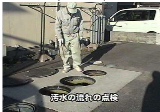
Checking inside the johkasou
