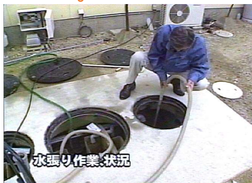
Filling the tanks with water
