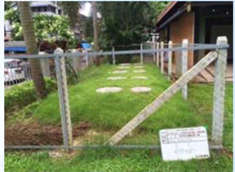
Johkasou installed in Maha Bandula Park (Johkasou capacity: 1.0 m 3 /d X 5 unit)
