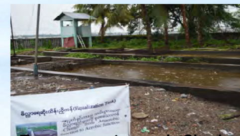
From septic tank Sludge treatment plant (dry-bed facility)
