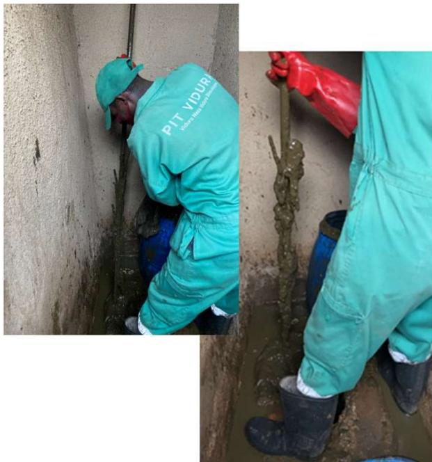
**Mechanical desludging without using vacuum car by PIT VIDURA (a private operator in Kigali City)**
