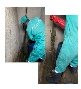
Mechanical desludging without using vacuum car by PIT VIDURA (a private operator in Kigali City)
