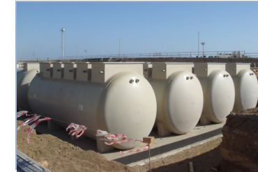
Employee dormitory (Saudi Arabia: 530m 3 /d)
