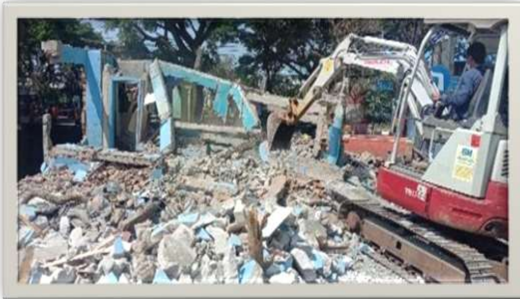
DEMOLITION OF ILLEGAL BUILDINGS
