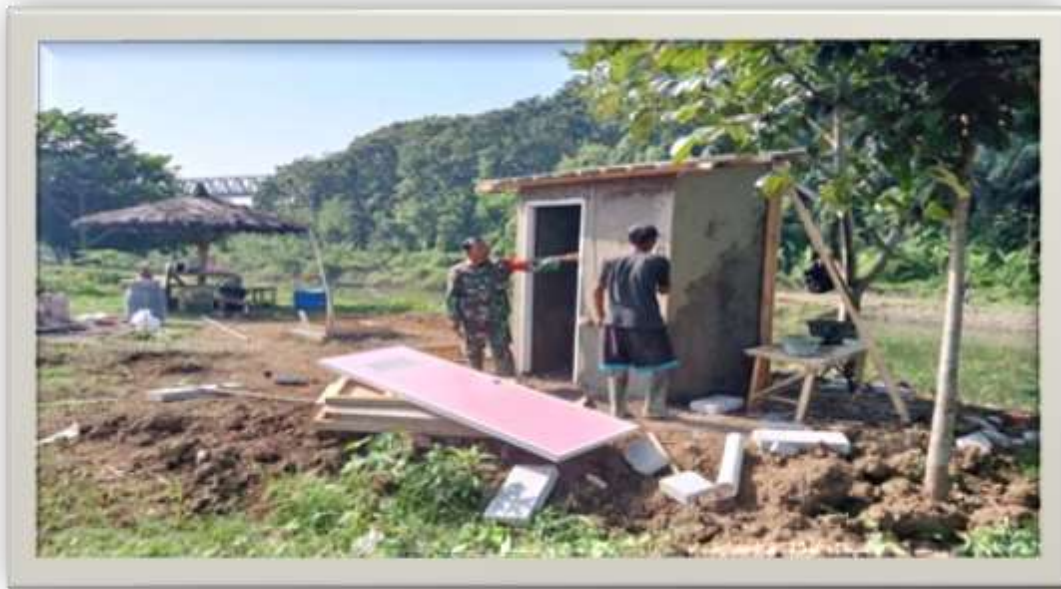
CONSTRUCTION OF COMMUNAL WC
