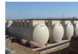
Employee dormitory (Saudi Arabia: 530m 3 /d)
