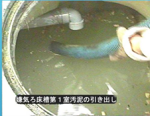
Drawing sludge out of the 2<sup>nd</sup>-room of anaerobic filter tank
