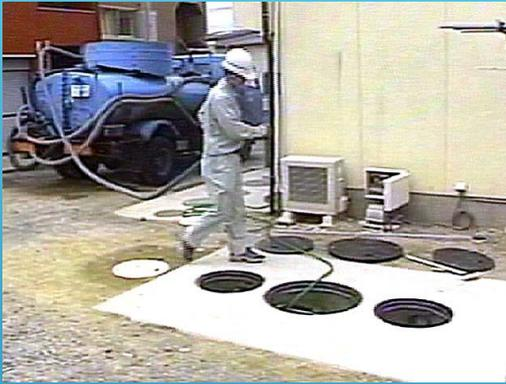
Drawing sludge out of the 1<sup>st</sup>-room of anaerobic filter tank
