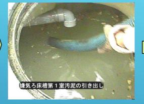
Drawing sludge out of the 2<sup>nd</sup>-room of anaerobic filter tank
